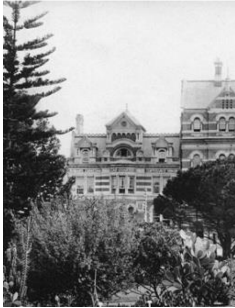
1897-98 Neil McNeil's Chambers, immediately south of Moir's Chambers by Talbot Hobbs in Barrack Street, Perth (007480d cropped)
