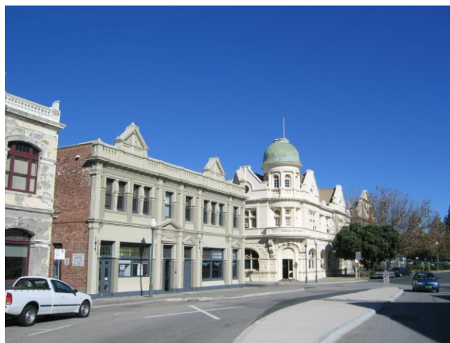
1898-99 office buildings for Neil McNeil on the south-east corner of Phillimore and Cliff Streets, Fremantle, with the Talbot Hobbs-designed Dalgety Buildings behind (John Taylor 2008)
